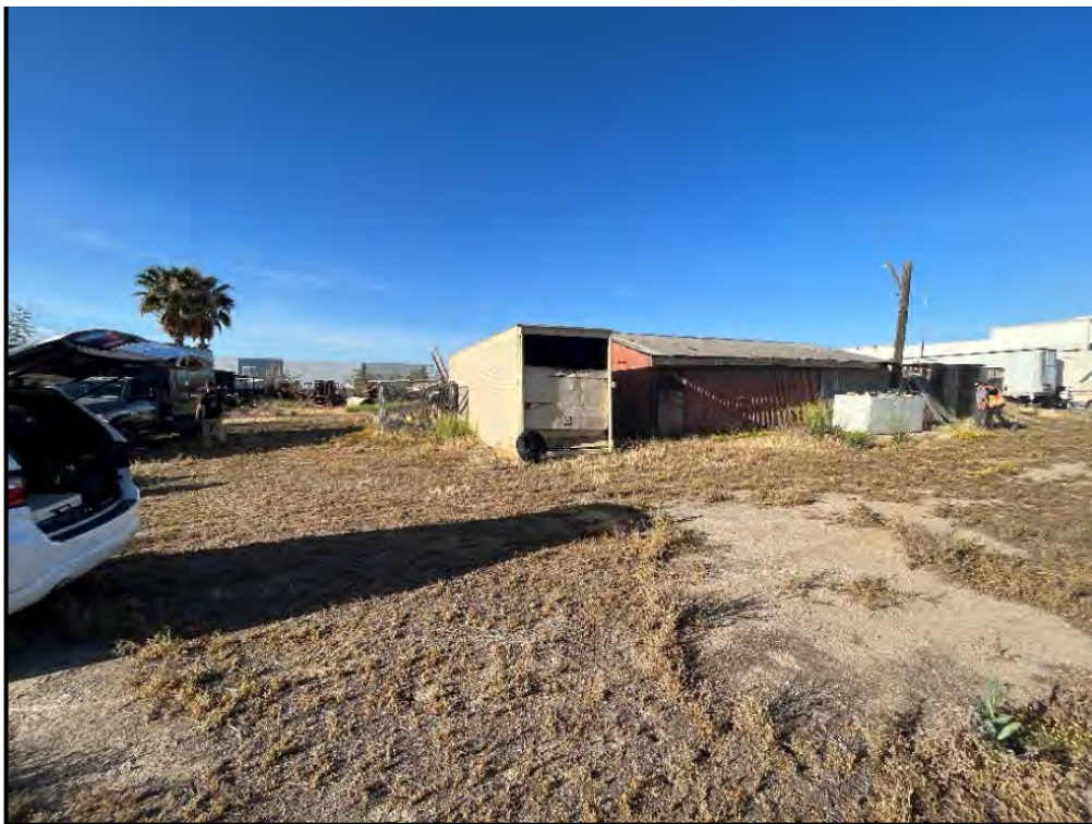
Plate 7: Overview of 995 West Markham Street and historic ancillary structure, facing south.
