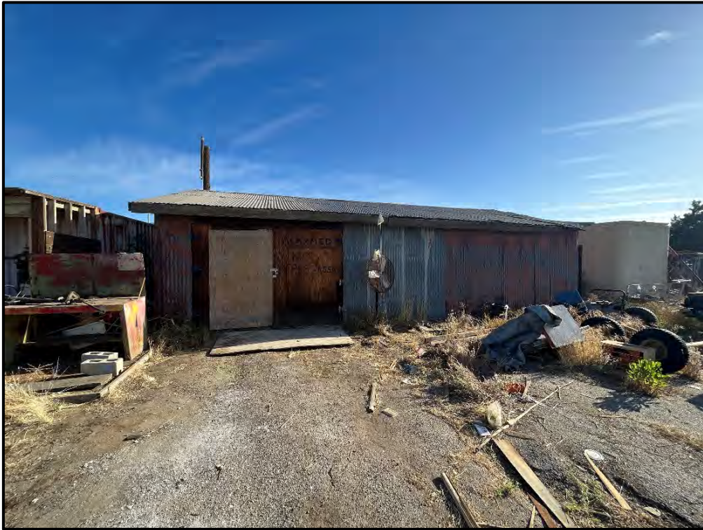
Plate 9: Southern façade of ancillary structure, facing north.
