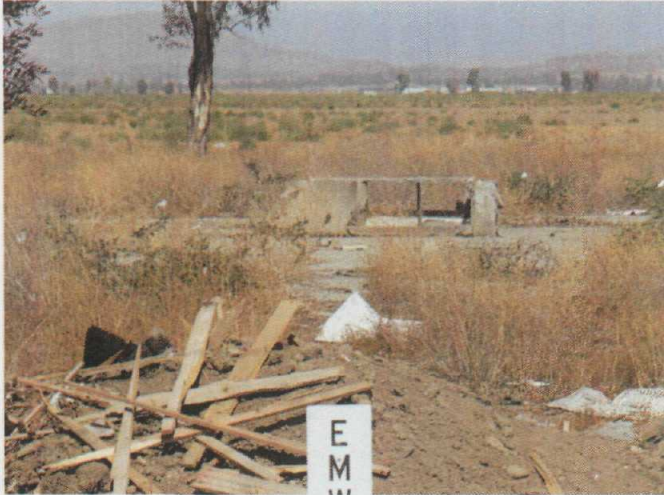
33-7705 Foundation overview, looking North
