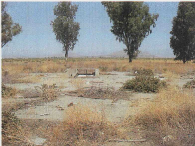
33-7705 Foundation overview, looking North
