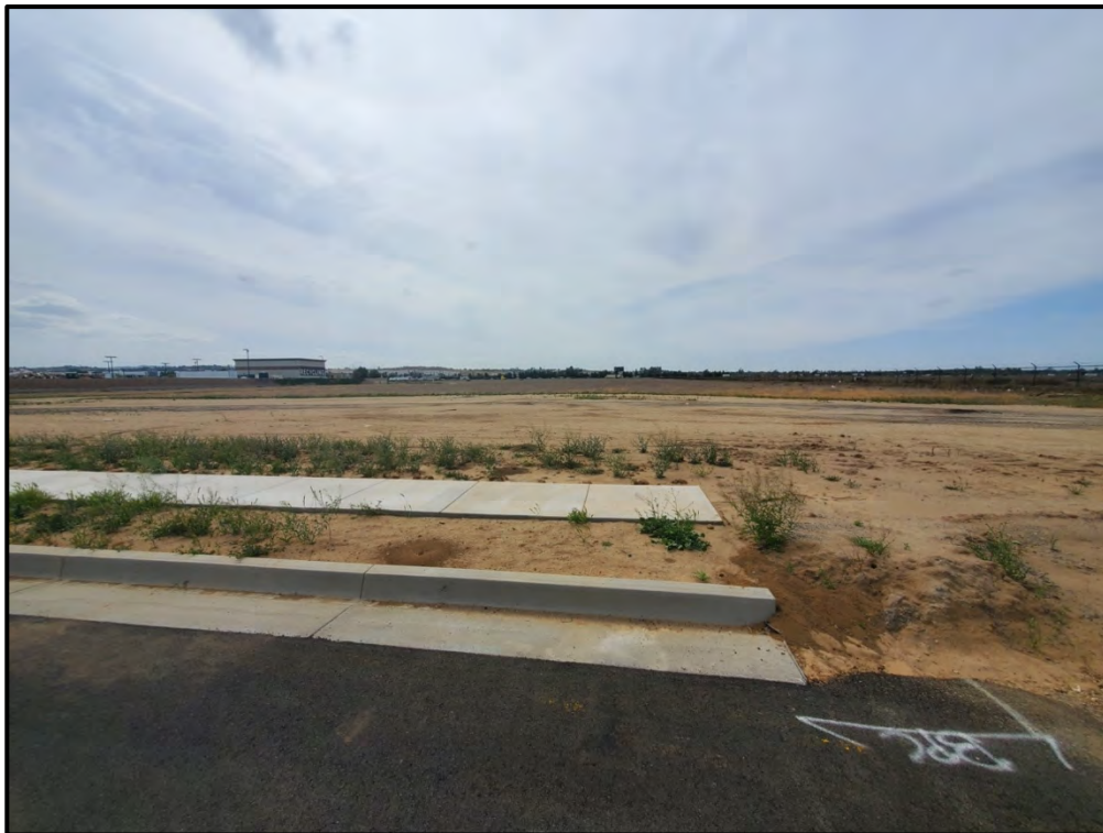
Plate 1: Overview of the western portion of the project, facing west.
