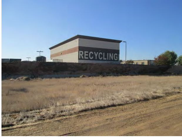
14. Southern adjacent recycling center buildings.
