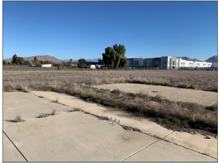
8. Small concrete foundations on the south central portion of the northern parcel, view facing east
