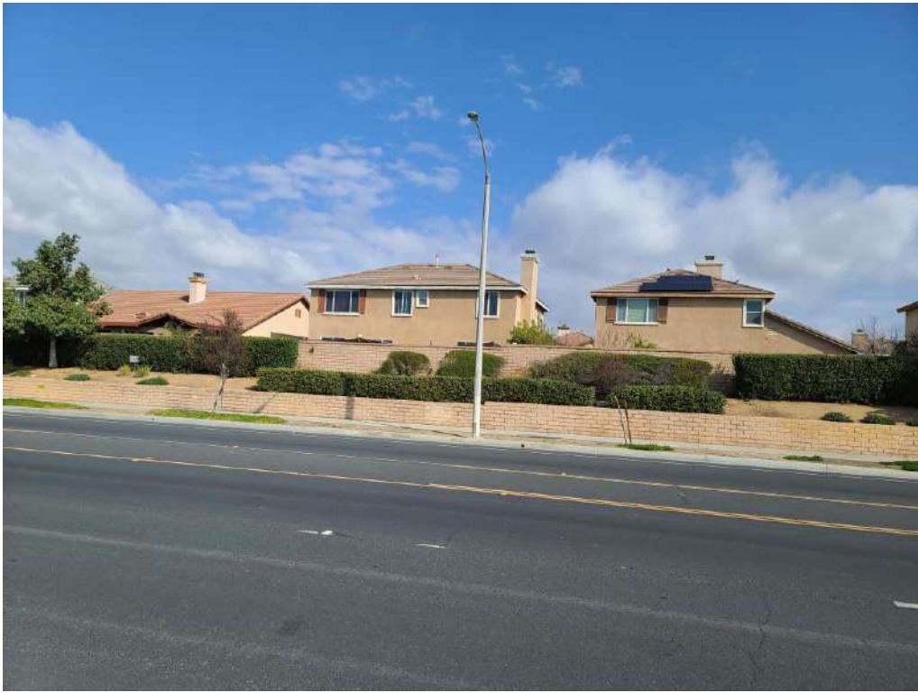
Photo 11: View of the adjoining property to the north.
