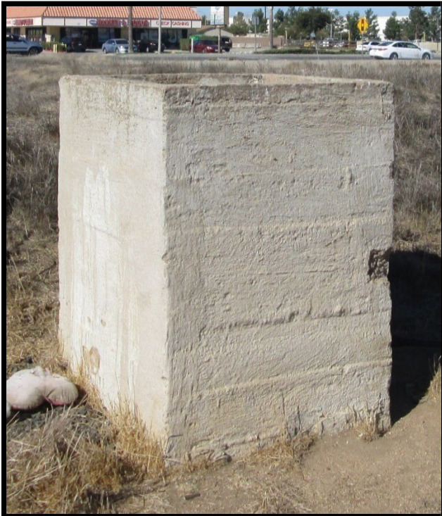
Square concrete standpipe.
