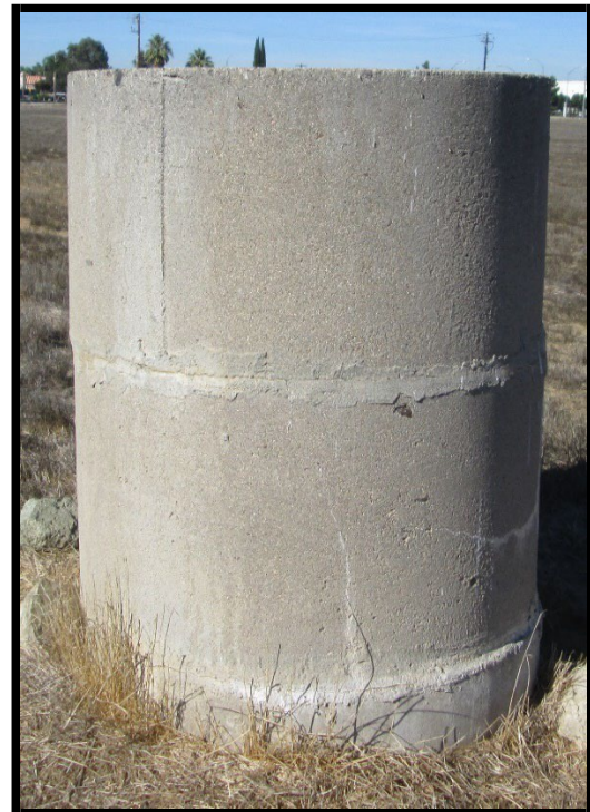
Cylindrical concrete standpipe.
