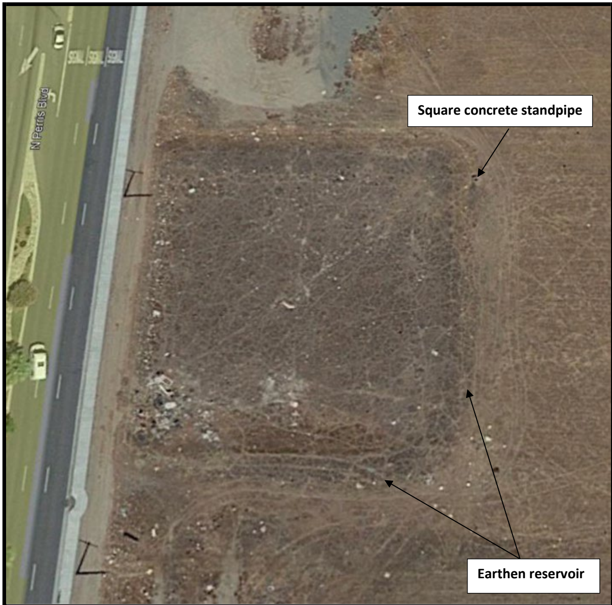
Figure 15: Aerial view of the earthen reservoir and square concrete standpipe originally recorded as P-33-008669. Adapted from Google Earth (August 2021).
