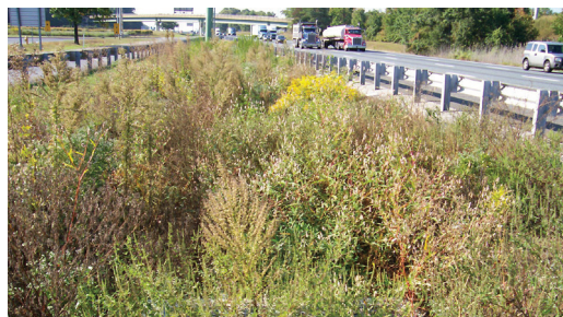
Bioretention facilities can provide food and shelter for potentially hazardous wildlife, but may be suitable with modification.
