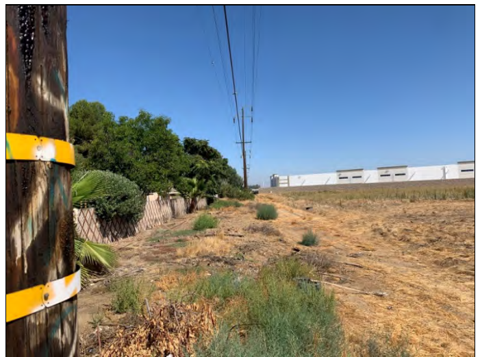
30. Electrical transmission lines on the western boundary, view facing northwest.
