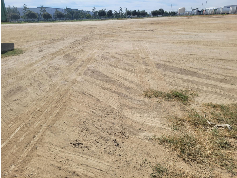
Figure 15: Evidence of Grading
