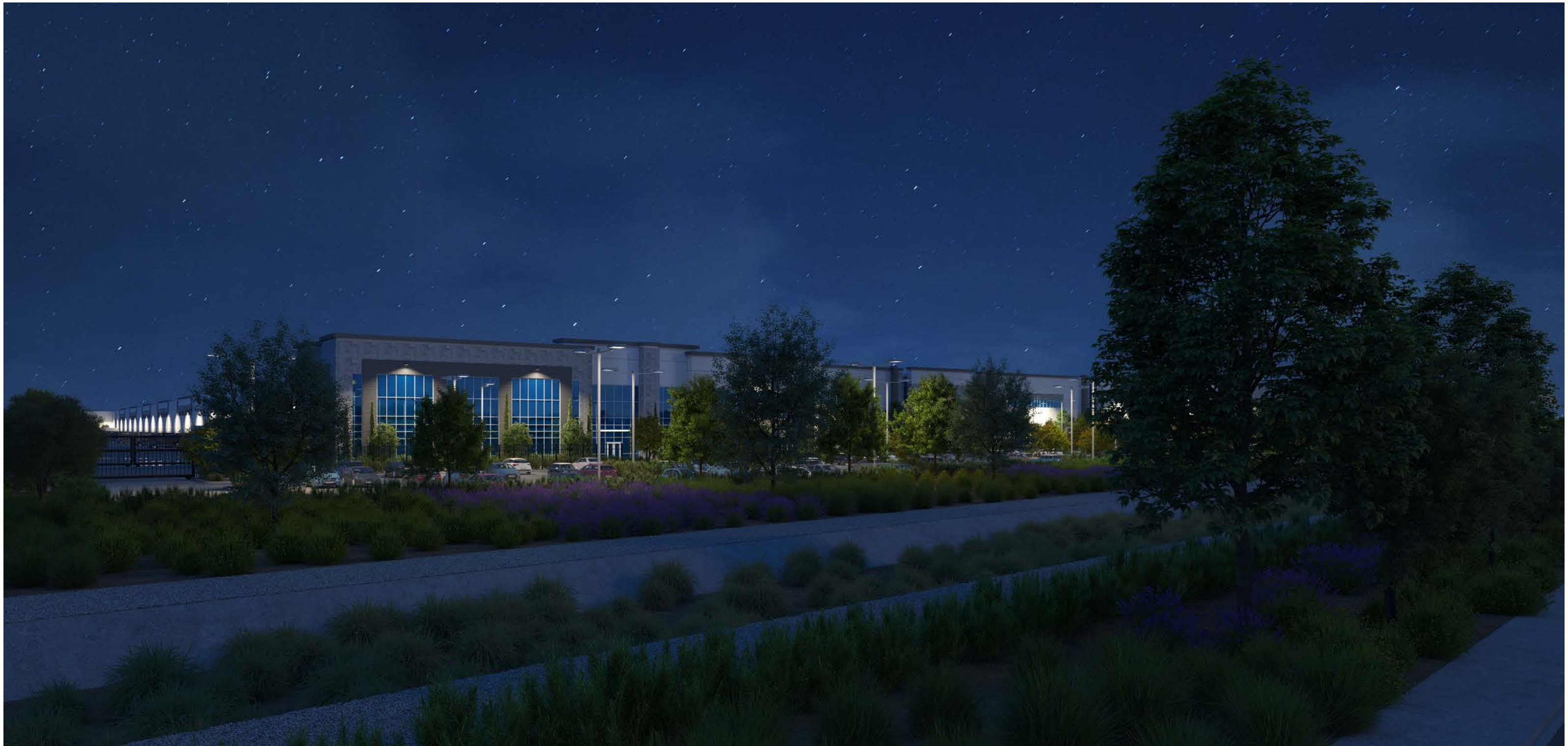
Night time perspective view from Watson St looking towards Building 2 from SW corner of the building
