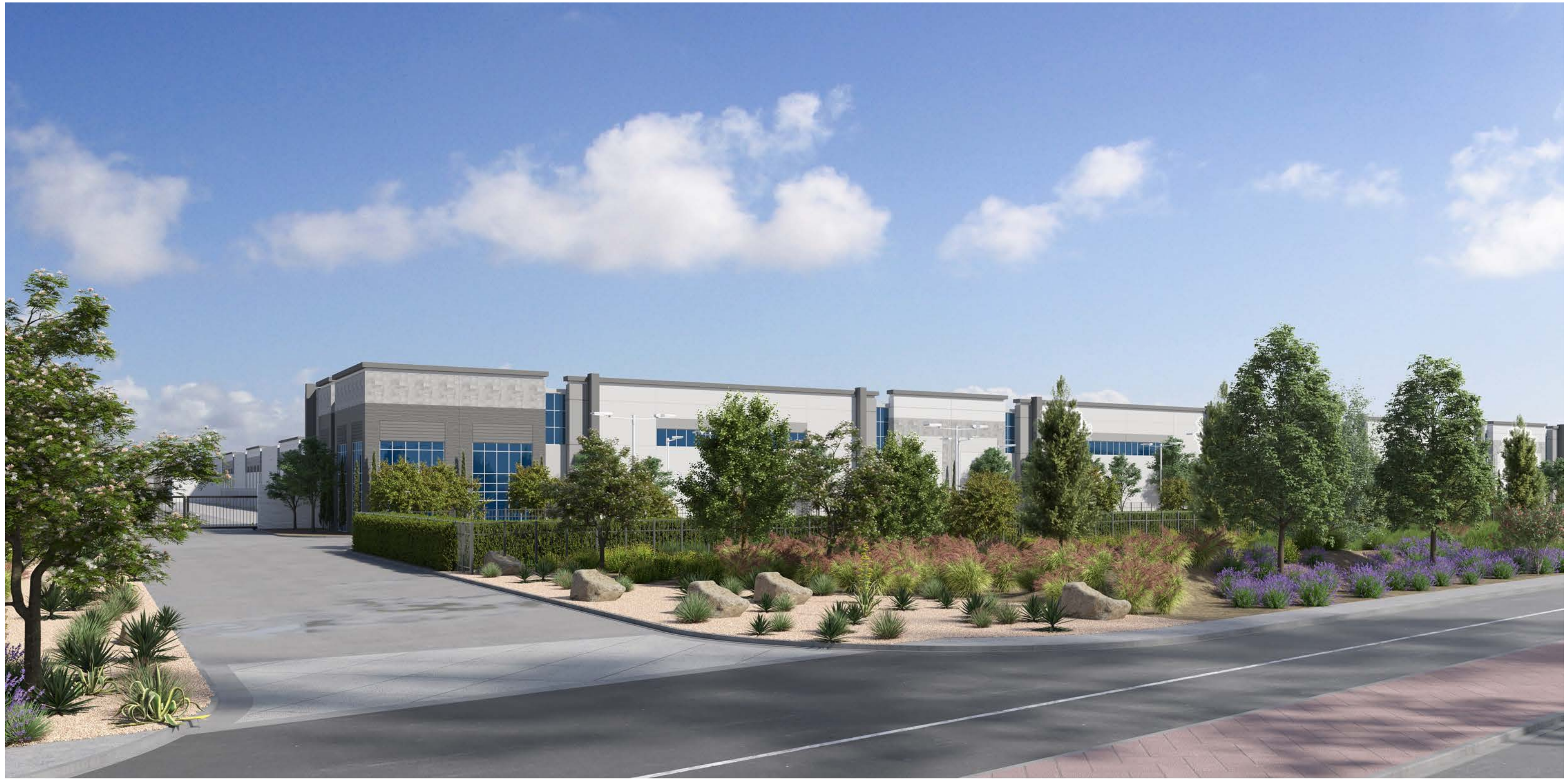
Perspective view from Mapes St looking towards Building 2 headed westbound
