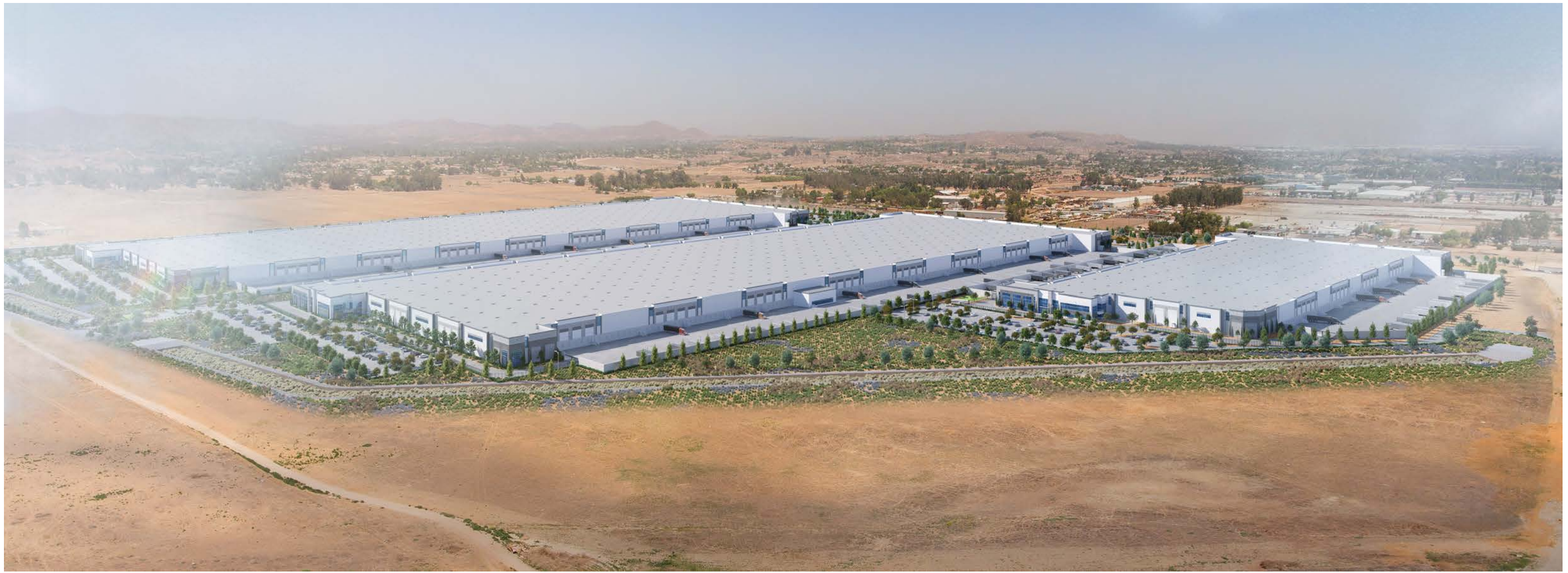
Aerial of final project from SE corner of the site.
