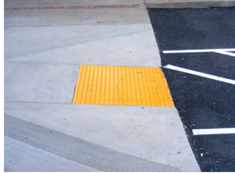
Truncated domes for Accessible needs
