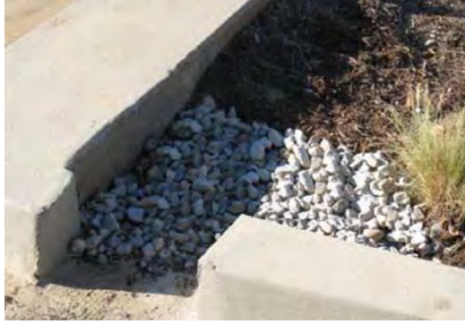
Figure 2: Curb Cut located in a Bioretention Facility
