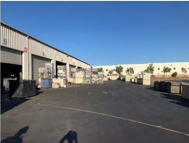
34. View of the operational area north of the 200 Sinclair Street building.
