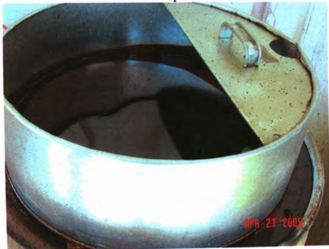
Waste oil from filter crusher
