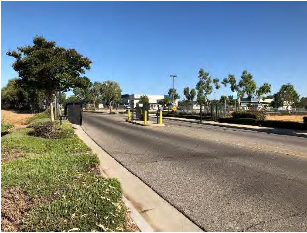
1. View of the Site entrance from Sinclair Street facing west-northwest.
