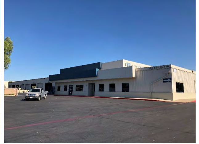
33. View of 200 Sinclair Street industrial building facing northwest.
