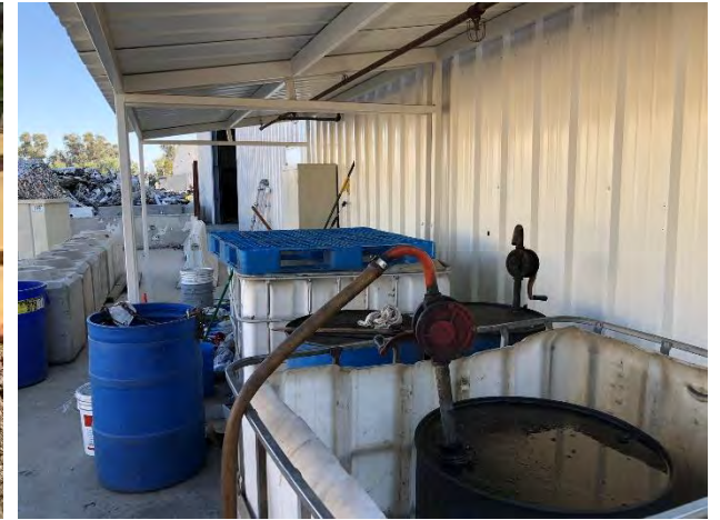
39. View of a 55-gallon diesel drum with plastic tote used as secondary containment.
