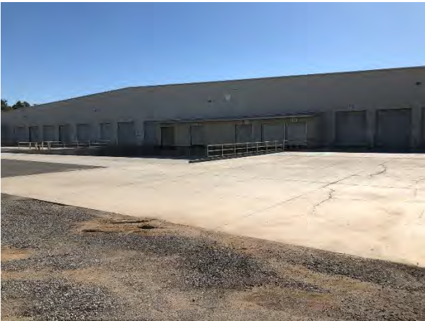
28. View of the loading docks on the west side of the 100 Sinclair Street building.
