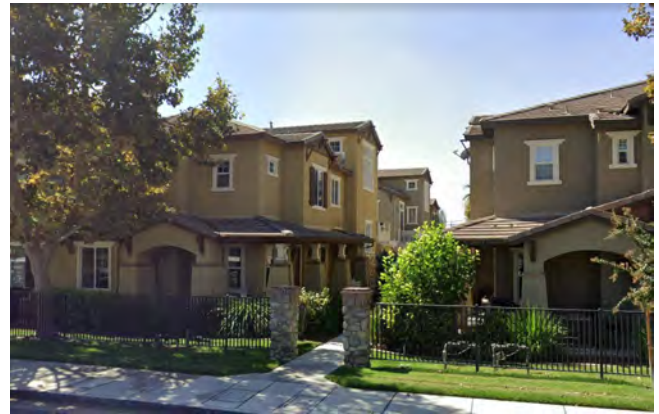
Standard 4.1 a. Setback design with a porch to create smooth visual transition from single family residential to multi-family.
