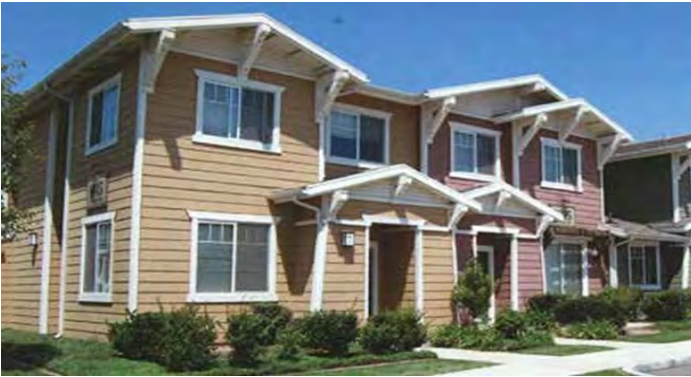
Standard 6.5.a: Rooflines should be broken at intervals no greater than 50 feet long by changes in height or step backs.
