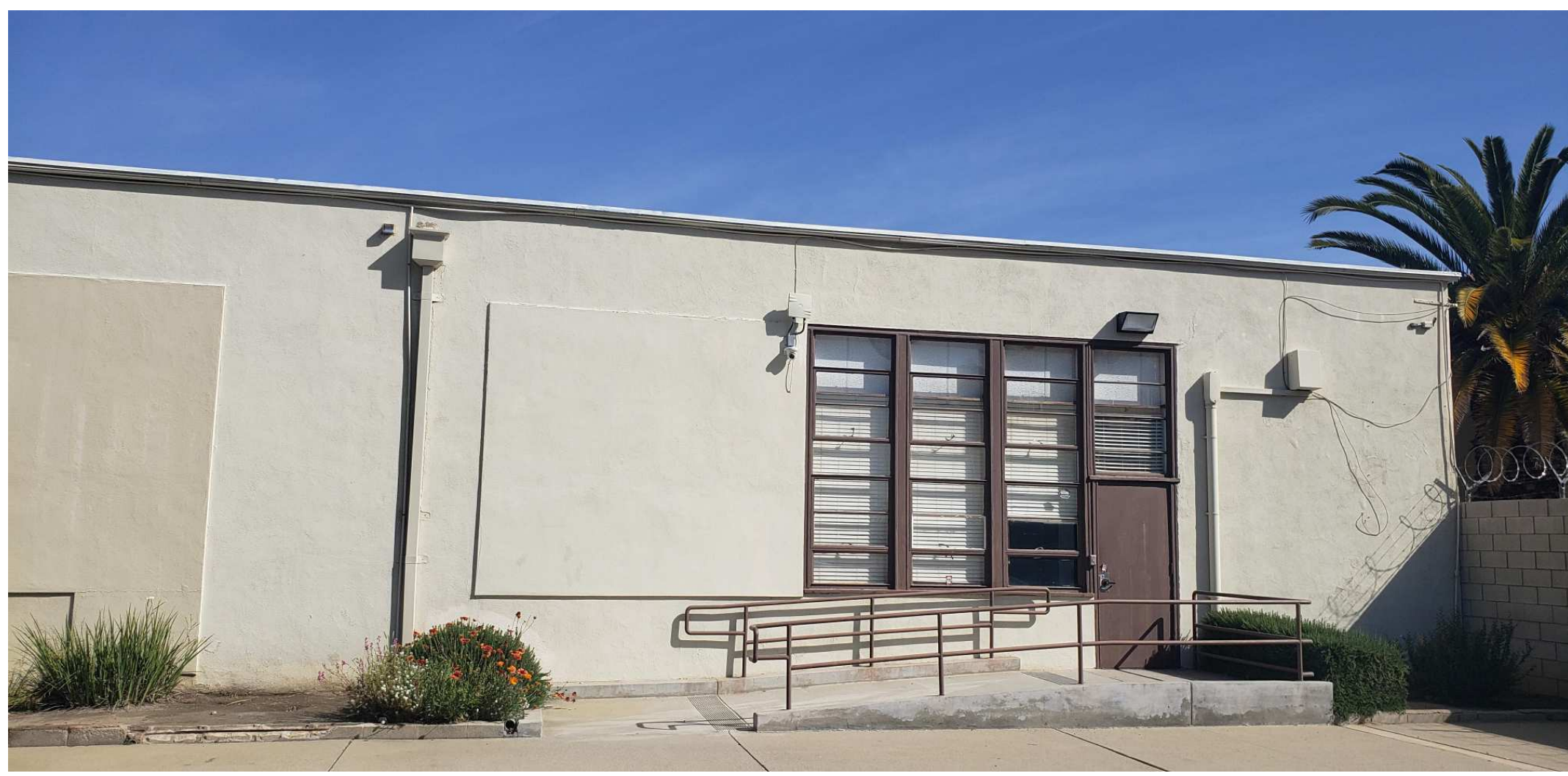
EXISTING ADA RAMP WITH (E) DETECTABLE WARNINGS
