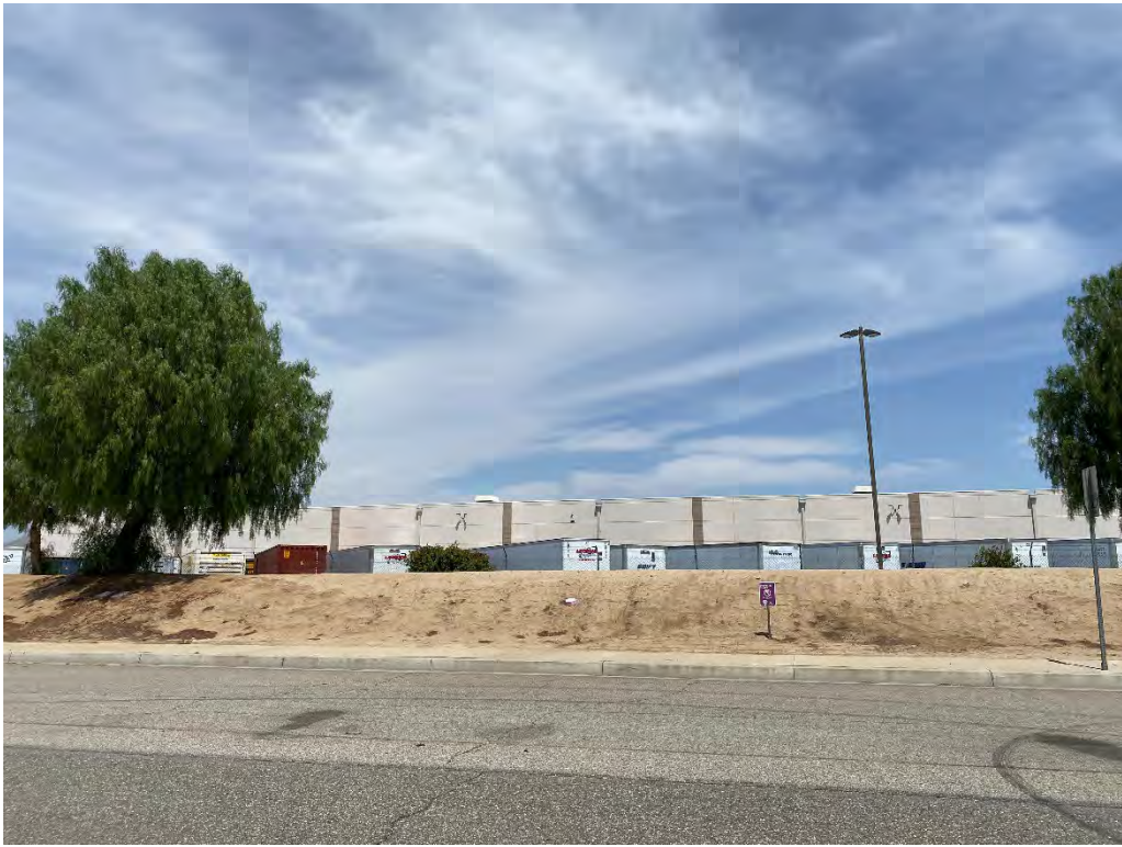
G-13. Adjacent distribution center to the east of Brennan Avenue (06/03/2022).
