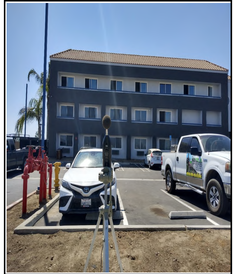
NM10 looking W away from S Redlands Avenue, across hotel parking lot, towards hotel building 480 S Redlands Avenue, Perris.
