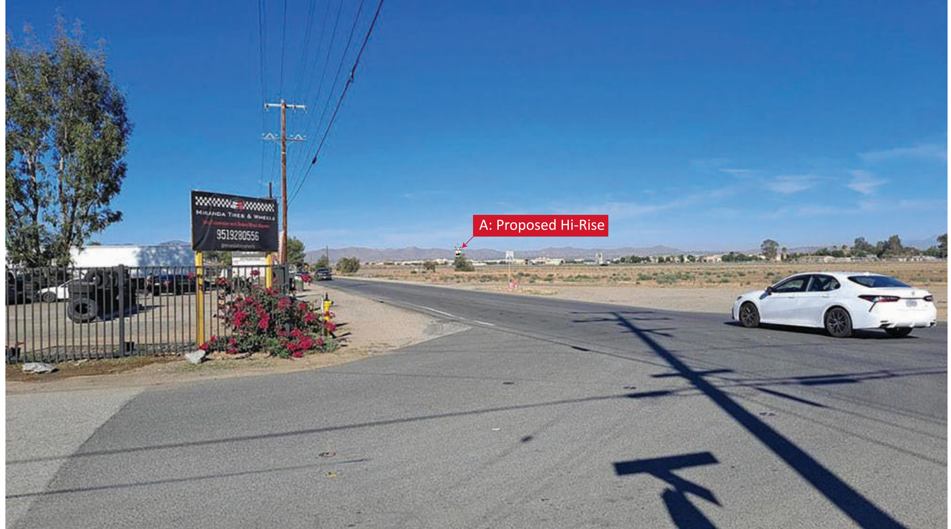
PHOTO VIEW LOCATION: CORNER OF ETHANAC RD. & TRUMBLE RD.
