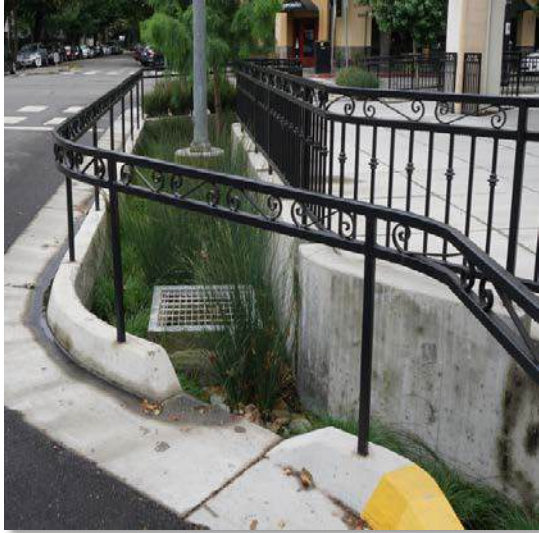
Figure A: Urban Infiltration Trench BMP
