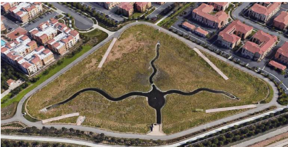
Figure A: Detention Basin BMP
