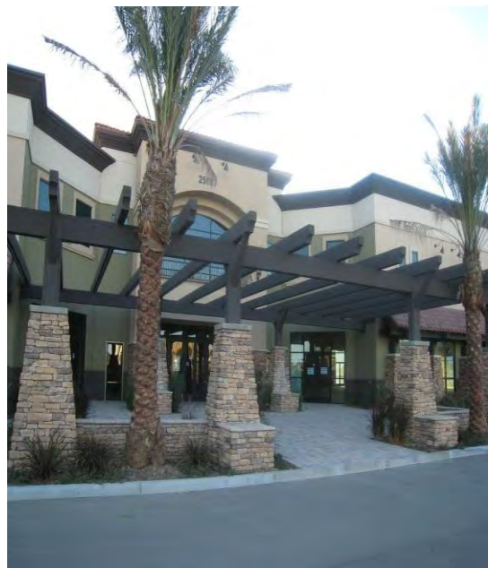
Building Entrances and Access Points
