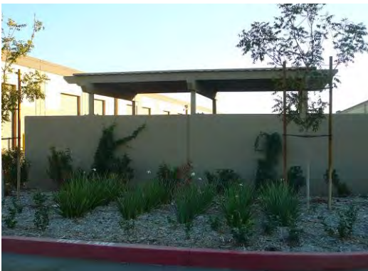
Covered Trash Enclosure
