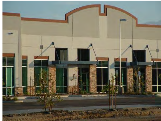
Roofs and Parapet
