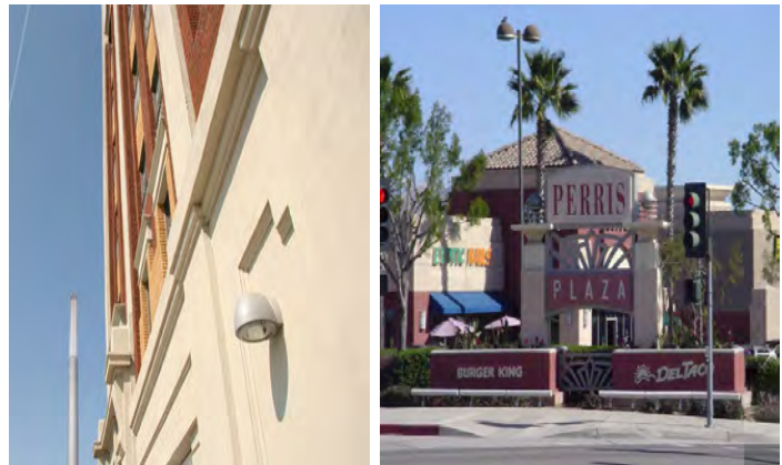
Lighting and Signage
