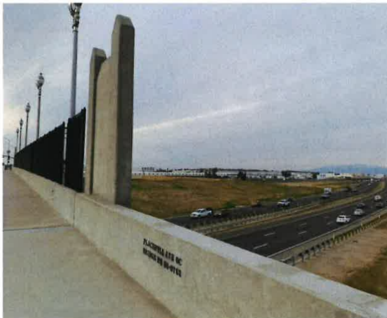
Figure 4 – Perris Valley Storm Drain
