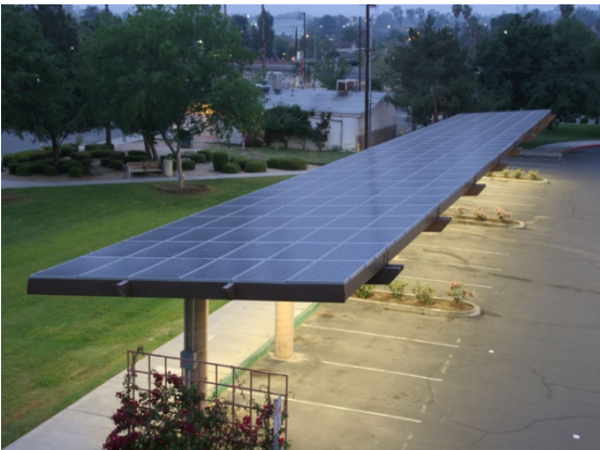
Perris Civic Center Solar Carports
