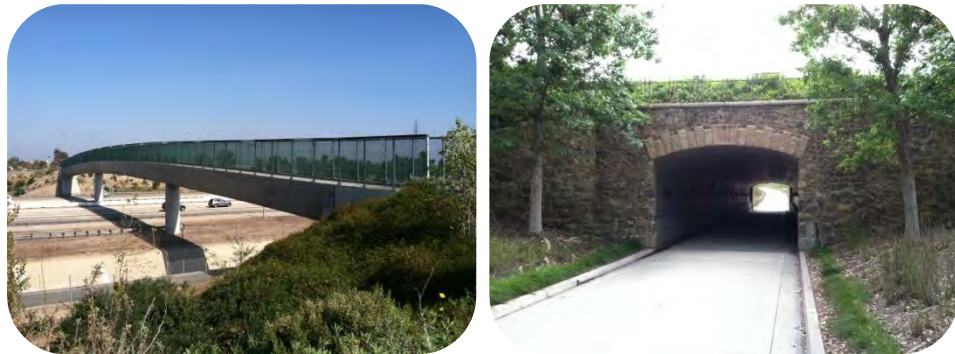
At-grade crossings over and under roadways.
