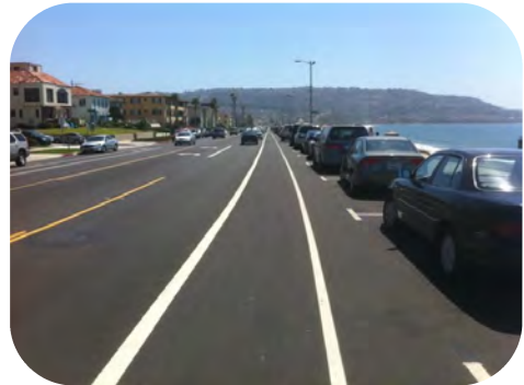
Buffered bike lanes with and without parking.
