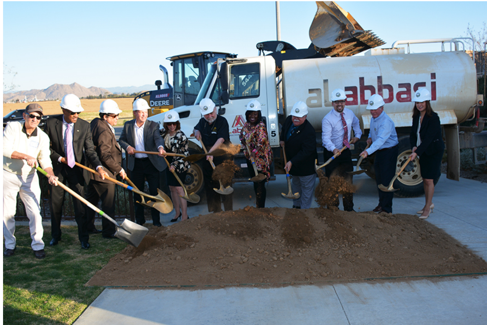
Perris elected officials and administrators join with colleagues from Menifee in the ceremonial ground-breaking for the Ethanac Road expansion in south Perris.
