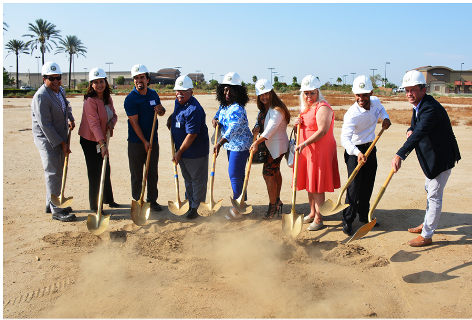
The City of Perris celebrated the ground-breaking August 21 for the Perris Plaza expansion. Dignitaries included City Manager Richard Belmudez, Assistant City Manager Clara Miramontes, Mayor Pro-Tem Malcolm Corona, Mayor Michael Vargas, City Councilwoman Tonya Burke, City Clerk Nancy Salazar, City Councilwoman Rita Rogers, City Councilman David Starr Rabb and developer Patrick Wood.
