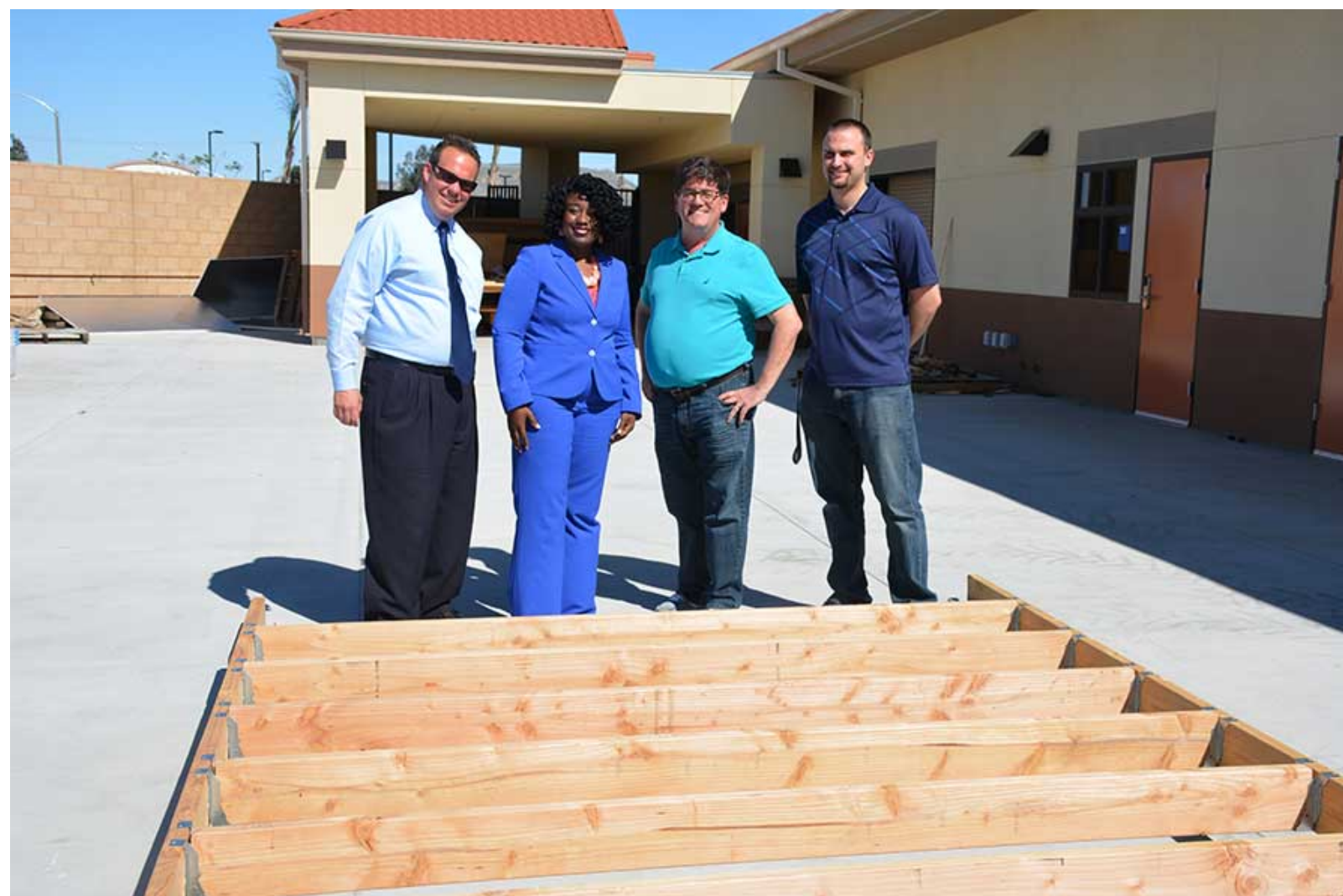
Perris City Councilwoman Tonya Burke stands in front of the foundation of a "tiny house" that one day may be donated to the City to house families needing shelter. With her are Orange Vista High School Principal Josh Workman, award-winning teacher Michael Towne and teacher Joe Russo.
