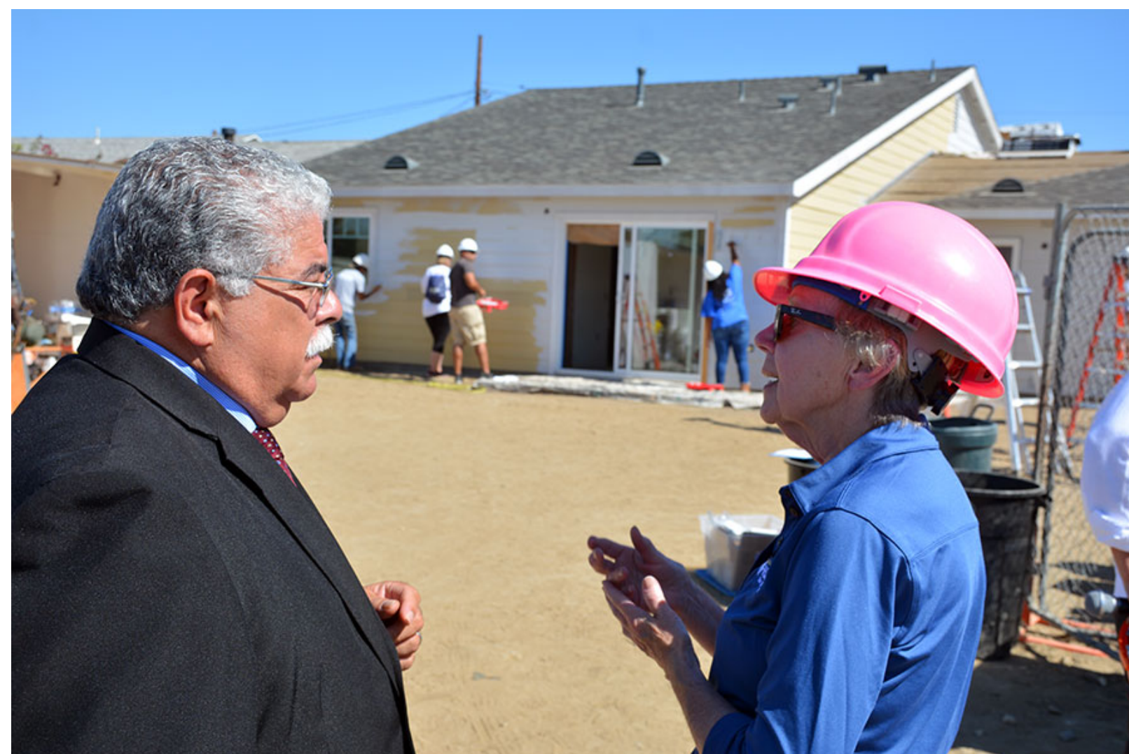
Perris Mayor Michael Vargas chats with Habitat for Humanity project manager Liz Bibb during a visit to the construction site on South Street in Perris, where two homes currently are under construction.
