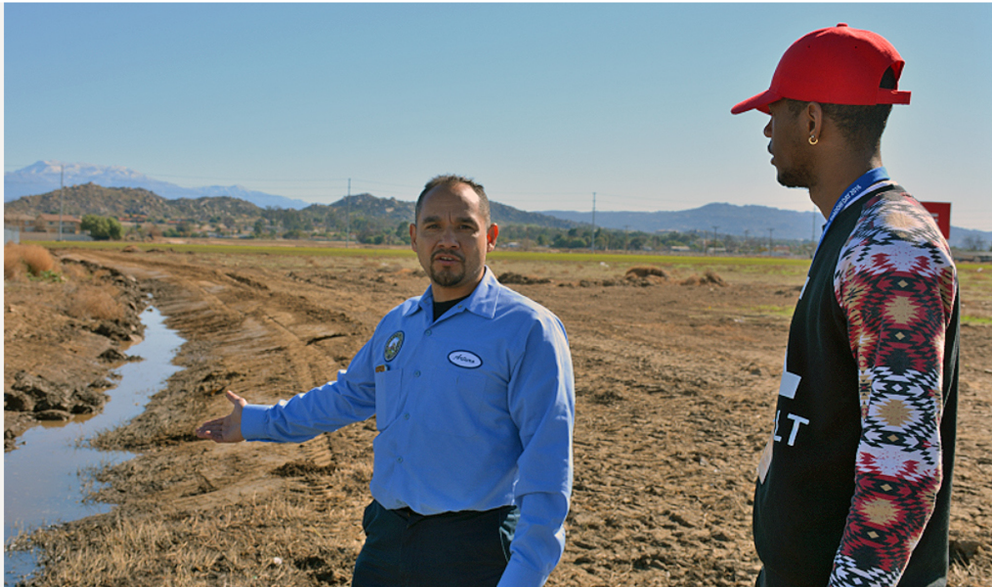
Public Works Supervisor Arturo Garcia shows a drainage ditch constructed by municipal employees to prevent flooding while Perris High School student Deion Martin looks on.
