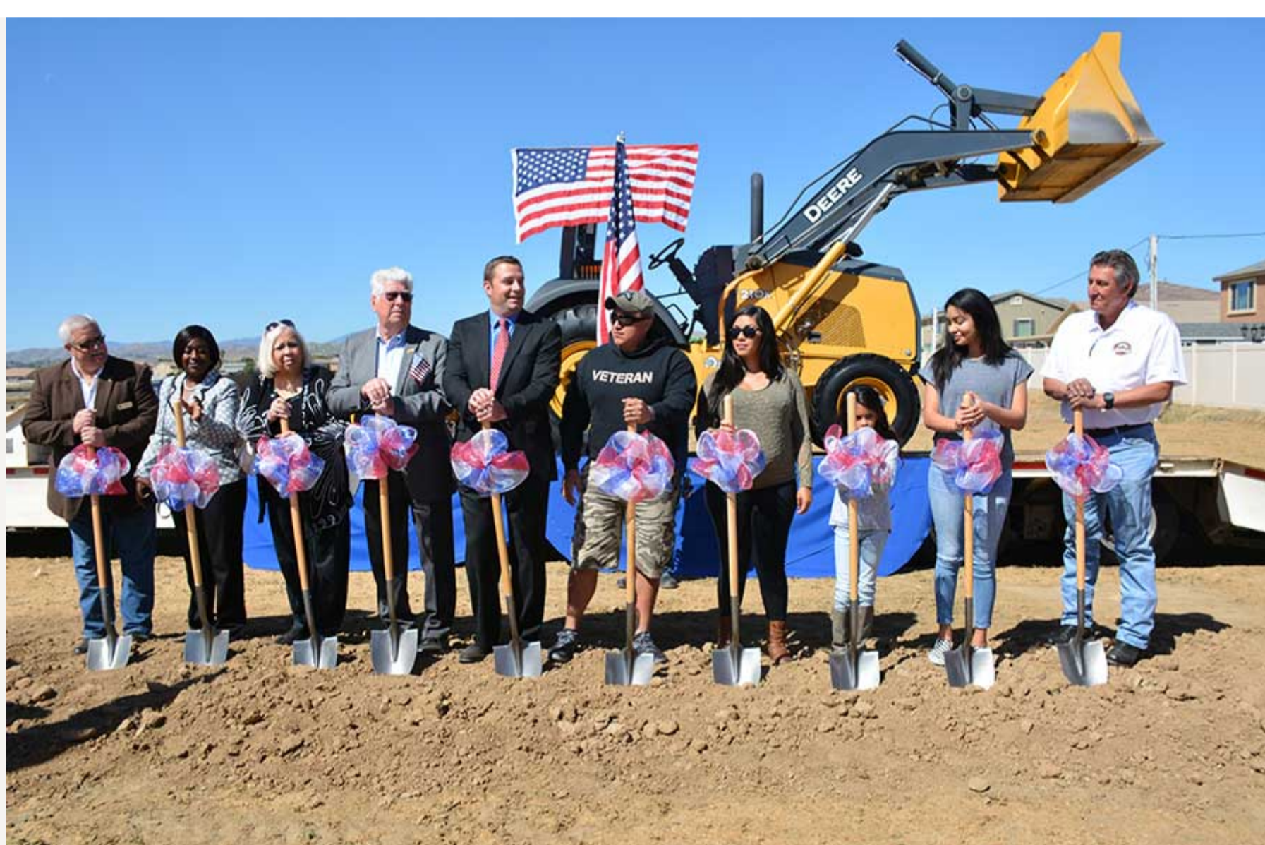
Perris elected officials join with Army Sgt. Oskar Zepeda and representatives from Pulte Homes to break ground at the site of the family's residence, scheduled for completion in August.
