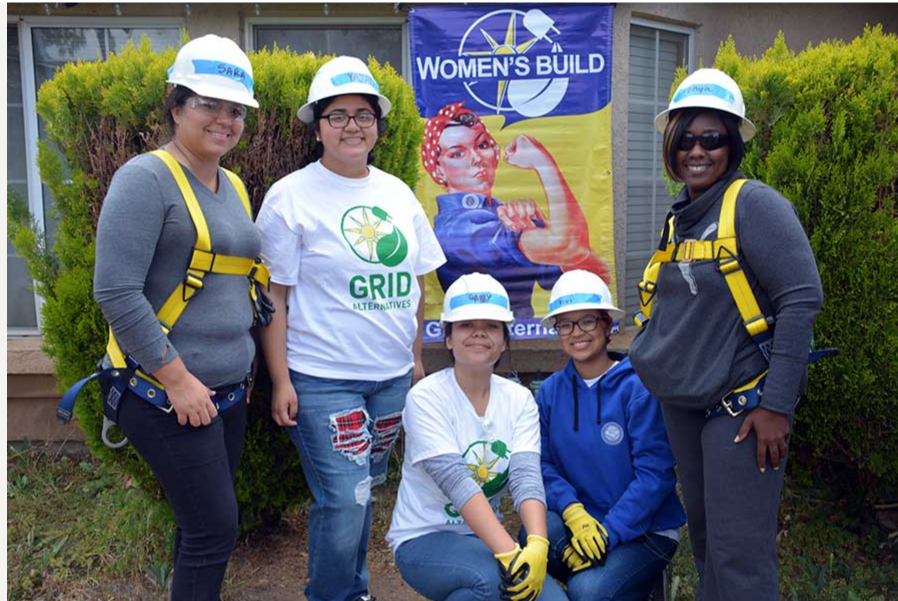
Sara Cortés-dePavon, who works in the City of Perris housing division, stands with Youth Advisory Committee members Yajaira Velazquez, Gabby Bulacan and Vivi Pavon-Cortés and Perris City Councilwoman Tonya Burke at the solar panel installation project May 7.
