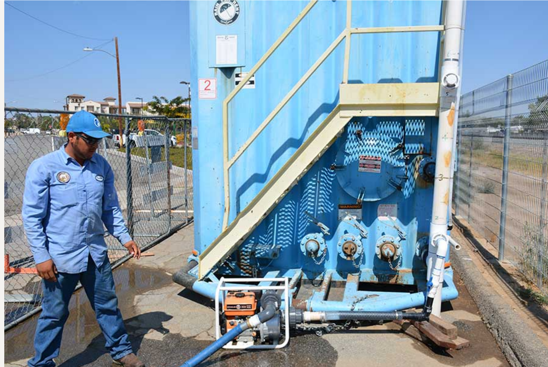
Perris Public Works employee Isauro Castillo watches as water is pumped from a 20,000-gallon tank to a portable tank for use at other City parks.
