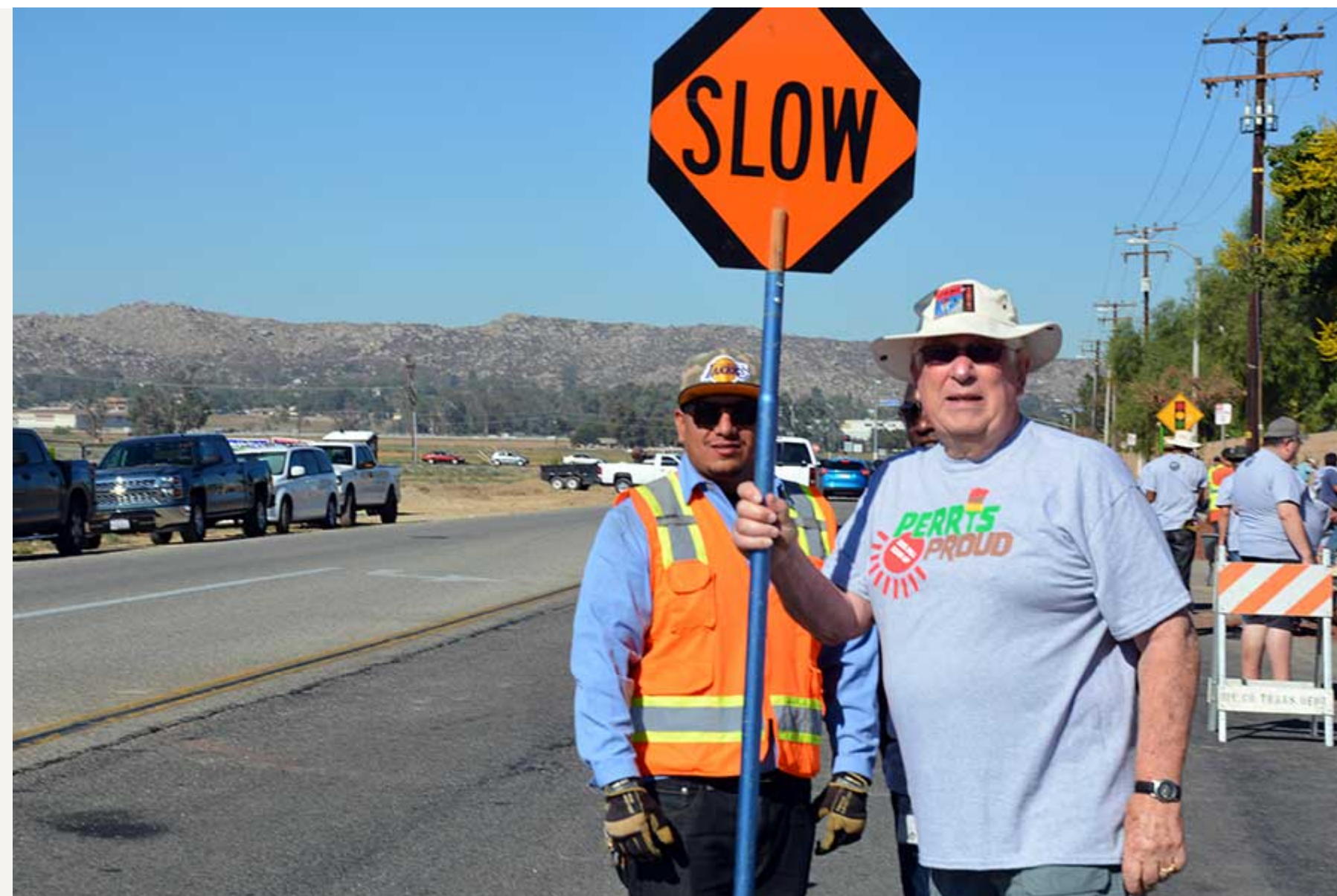
Perris Mayor Daryl Busch holds a sign to slow traffic through the work area.
