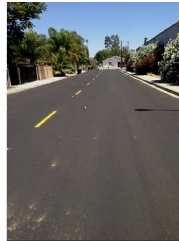
Images of Park Street, north of South Boulevard, show before and after results of applying a of slurry seal to prevent further road deterioration.
